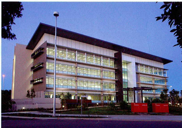
Both small and large airports can benefit from property development partnerships. (Gateway)
