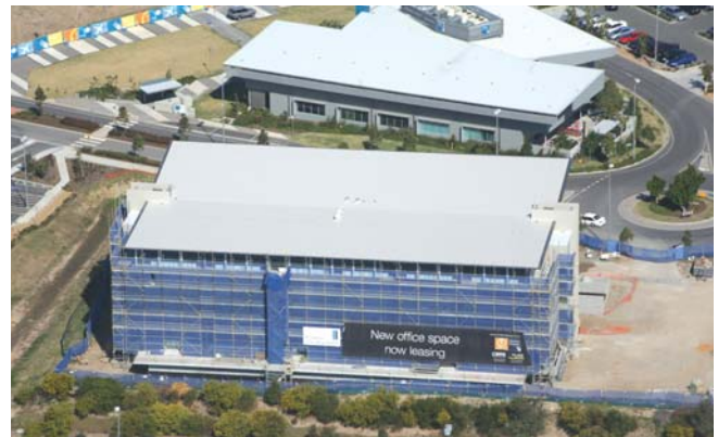
Gateway Project Partners has partnered with Brisbane Airport Corporation on the Airport Drive development. (Gateway Project Partners)
